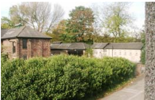
Photograph 5: Main courtyard area (1)
