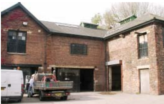
Photograph 6: Main courtyard area (2)
