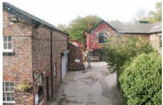
Photograph 9: Courtyard 2003: Access route and toilets/gardeners area
