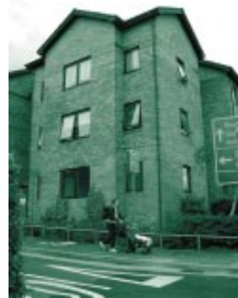
This building is designed with windows on both the front and side elevations so as to afford good surveillance
