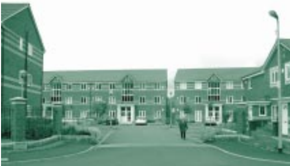
Semi private zone demarcated by a change in road surface along with symbolic pillars and railings.
