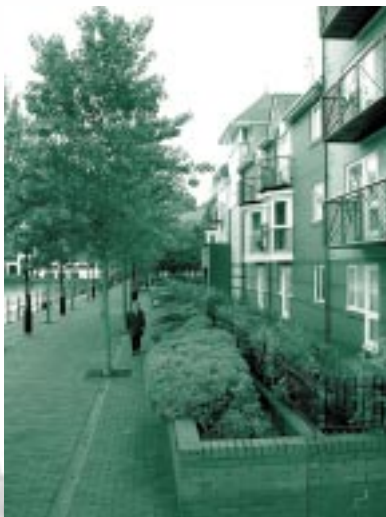
A low wall with railings on top makes for a well defined private space. Low lying shrubs provide an extra buffer.
