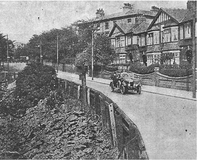
Below: Landslip top of Lower Broughton Road 1920s
