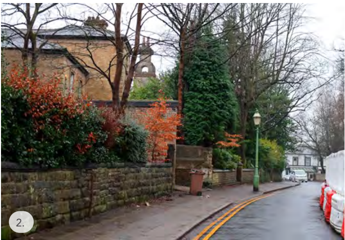
View 2: View down from the top end of Lower Broughton Road capturing the topology of the area and drawing the eye towards the historic properties that line the road.
