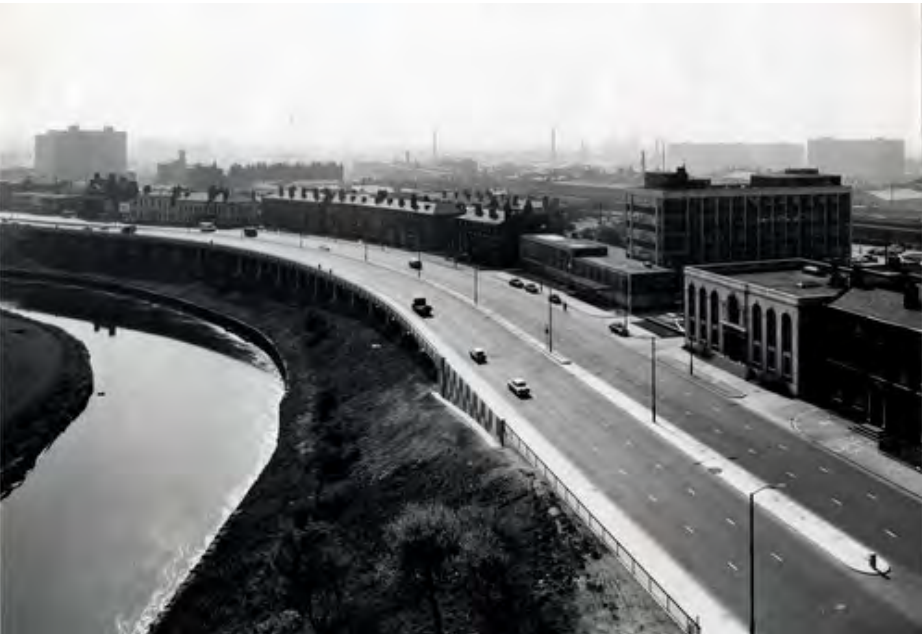
Figure 4 A6 Crescent widening, completed. Photograph taken from roof of R.C.A.T. at 10.15am on 12 May 1965
